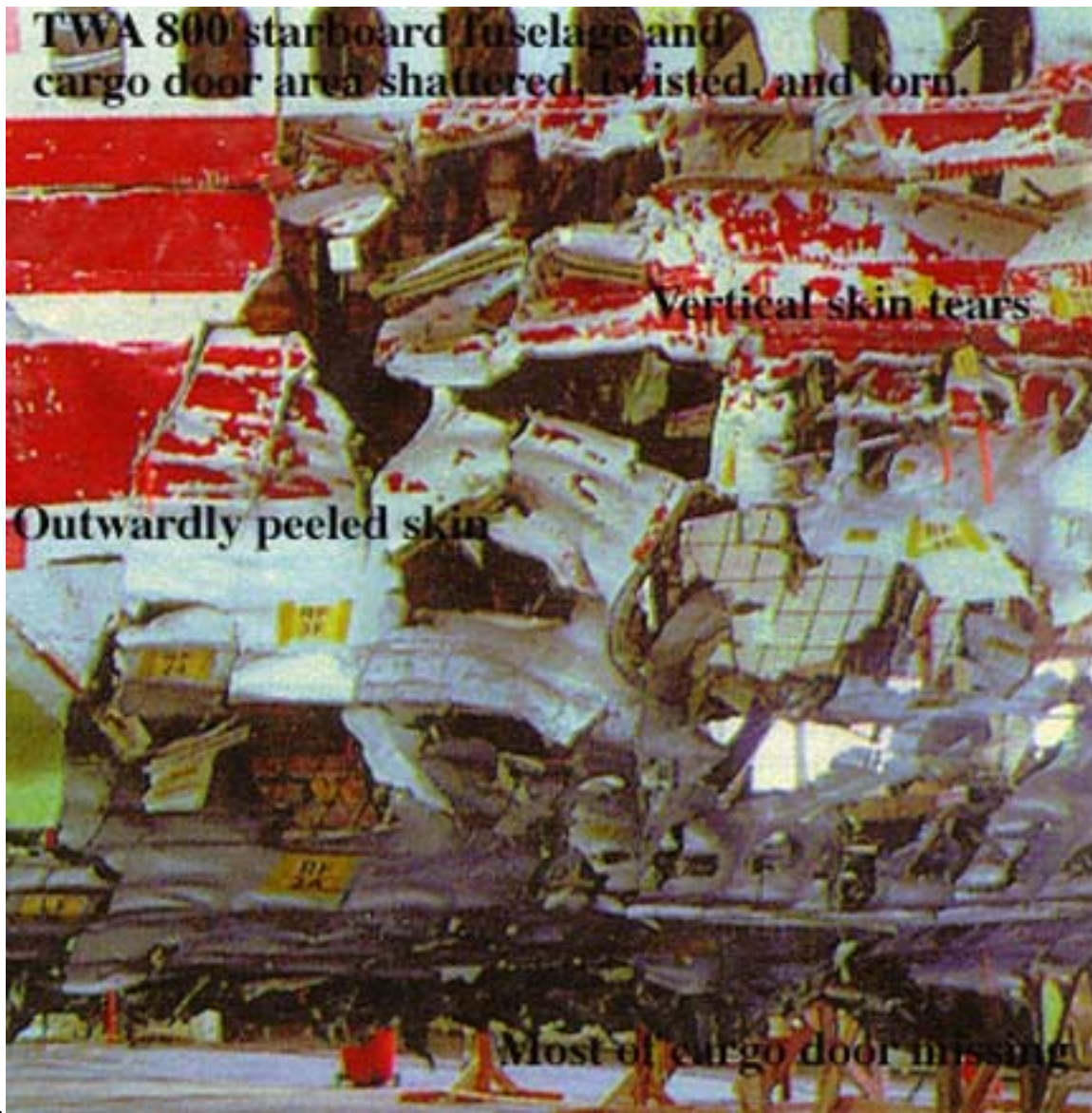
Caption for above photograph: Shattered starboard side around forward cargo door of Trans World Airlines Flight 800 revealing outwardly and petaled shaped skin around aft midspan latch.
